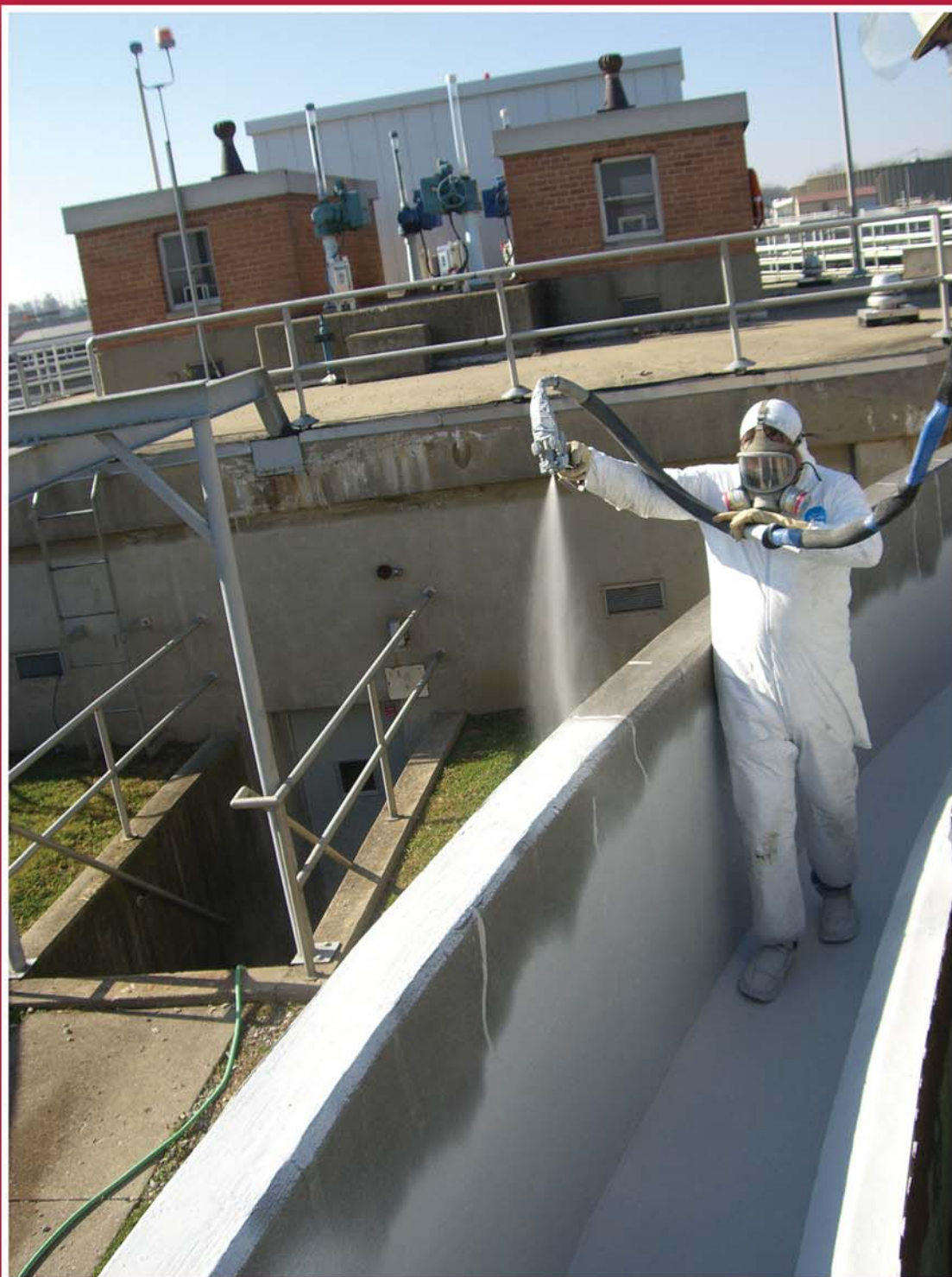
Pure Polyurea coating applied to secondary containment at a water treatment facility
