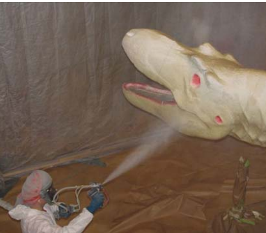
Polyurea Coating sprayed on foam and EPS
